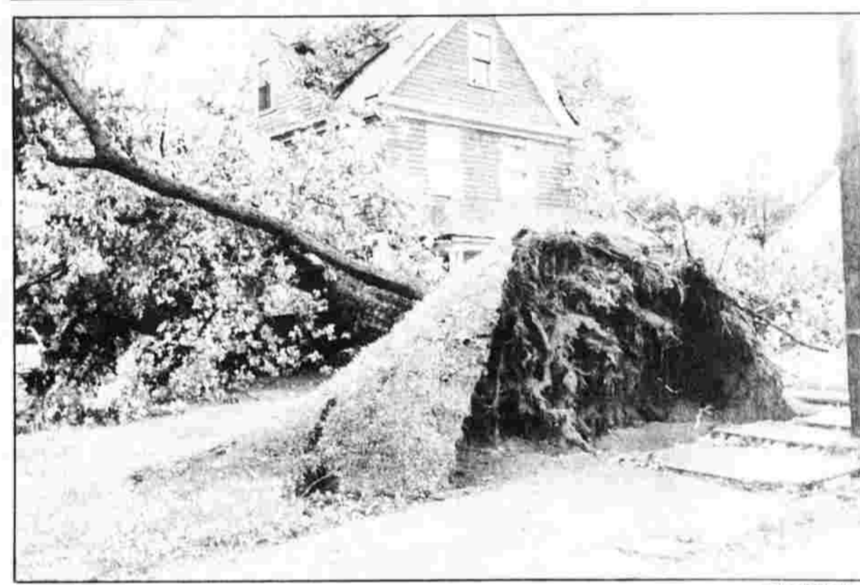
LOOKING BACK — A sample of the damage caused in 1985 by Hurricane Gloria.
